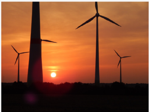
Golden Hills North Wind Energy is located in Eastern Alameda County, and is expected to be operational at the end of 2017.
