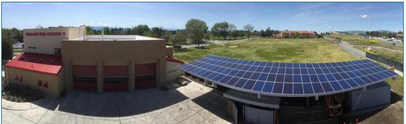
Figure 29: Aerial view of the Fremont Fire Station 11 Microgrid, a model for advanced emergency services microgrids and enhanced community resilience through innovative clean energy applications- developed by Fremont-based Gridscape Solutions.
