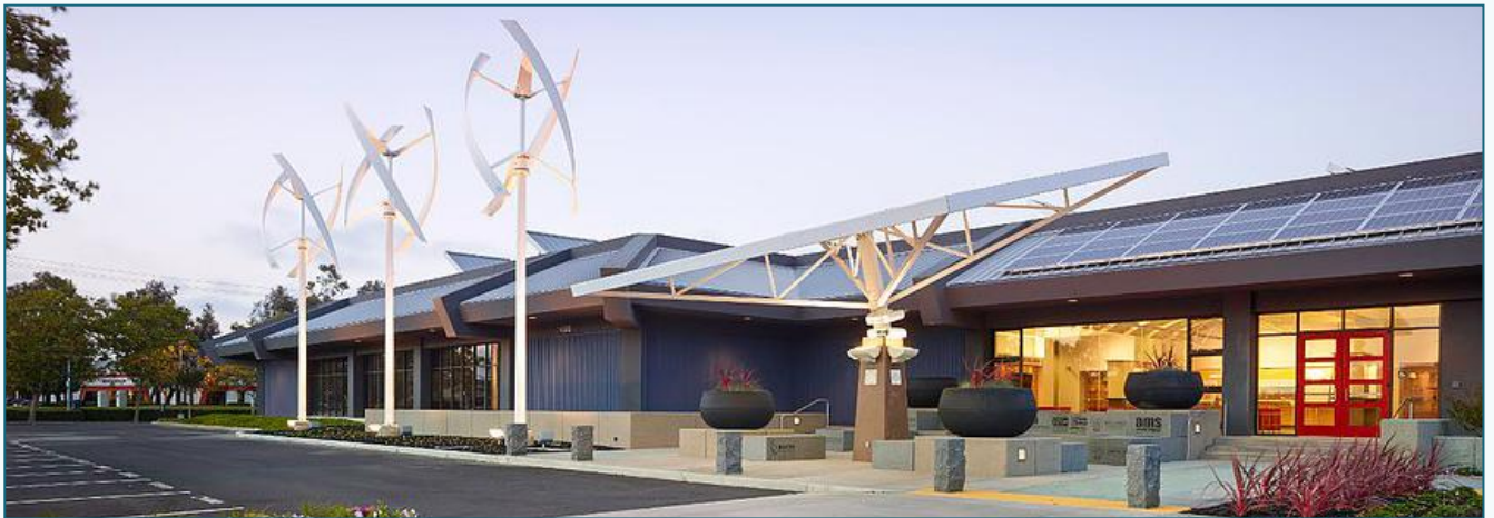
Figure 28: Front view of the IBEW 595 Zero Net Energy Center in San Leandro, which was designed to be a world-class example of a ZNE building.
