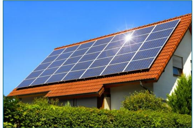
Figure 4: Rooftop residential solar is a common application of NEM.
