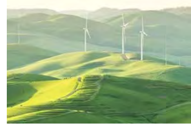
Mulqueeney Wind Project
