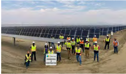
Rosamond Central Solar Project
