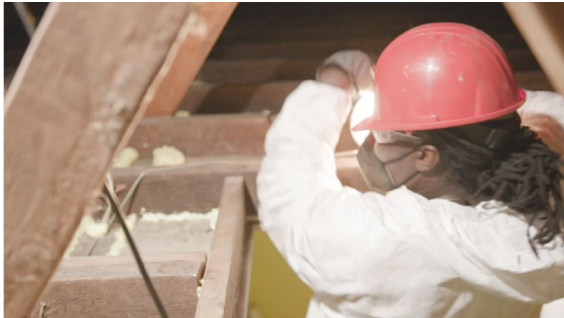
Pictured: Reymon Lacheaux, homeowner (above); worker with Eco Options (below) Source: Elemental
