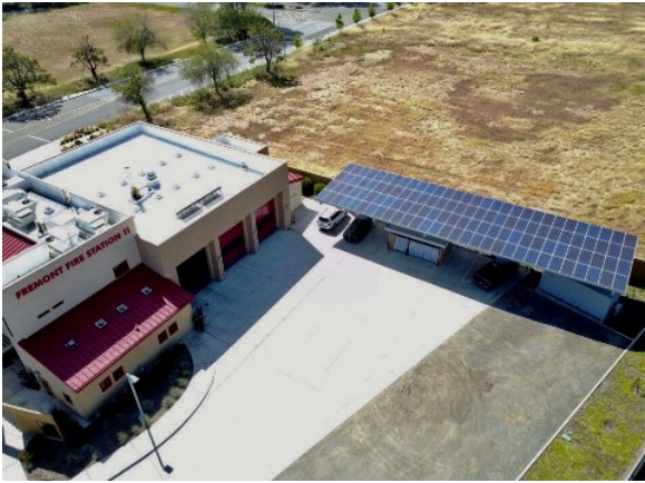
Fremont Fire Station Microgrid
