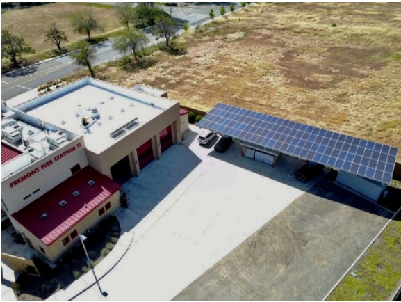
Fremont Fire Station Microgrid
