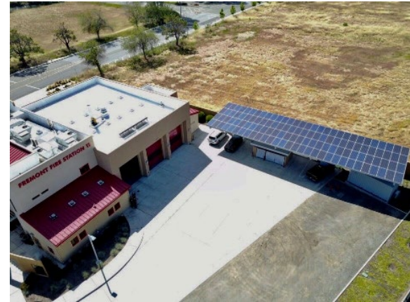
Fremont Fire Station Microgrid
