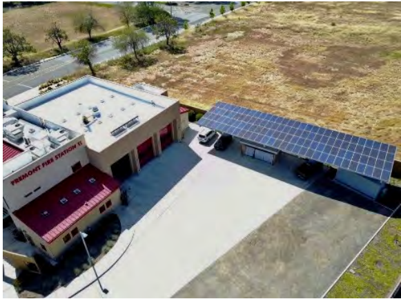
Fremont Fire Station Microgrid
