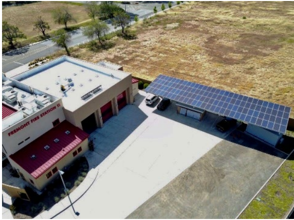
Fremont Fire Station Microgrid
