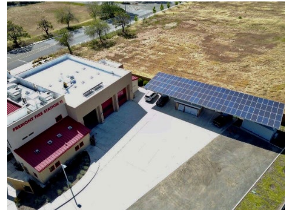
Fremont Fire Station Microgrid
