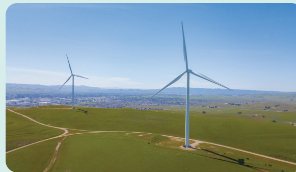
The Scott Haggerty Wind Energy Center, an Ava power project, is located in Livermore, CA and produces enough electricity to power over 47,000 homes.
