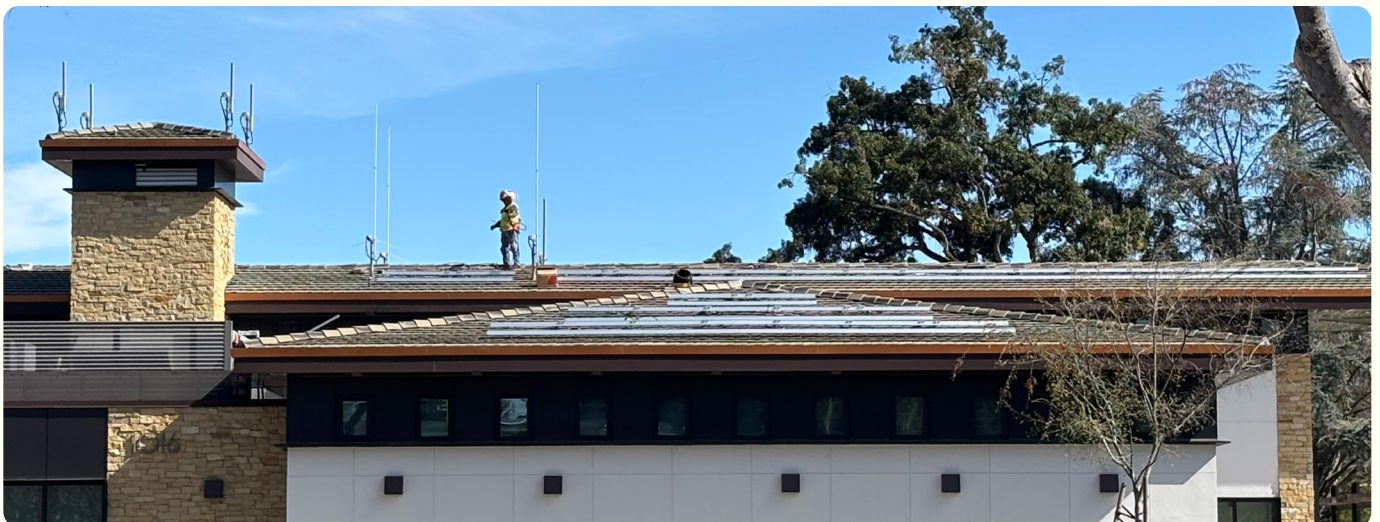
Photovoltaic (PV) solar panels being installed on the roof of the Livermore City Council Chambers.
