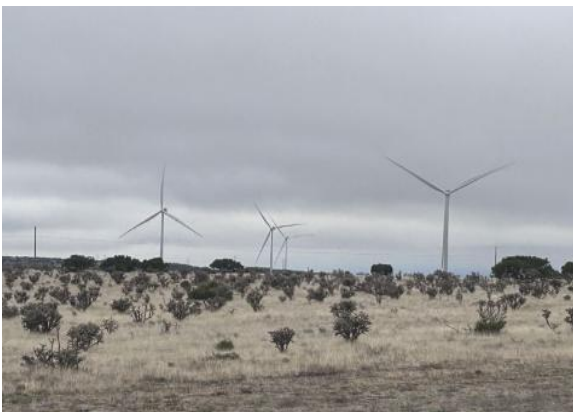
1 SunZia North wind turbines, Lincoln County, NM
