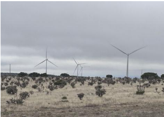
1 SunZia North wind turbines, Lincoln County, NM
